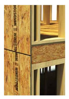
Engineered Wood Association, which rates and certifies structural sheathing products for construction. The panels strengthen what is essentially a bunch of nails used to fasten the framing members at that critical joint to make the house considerably stronger and safer.
