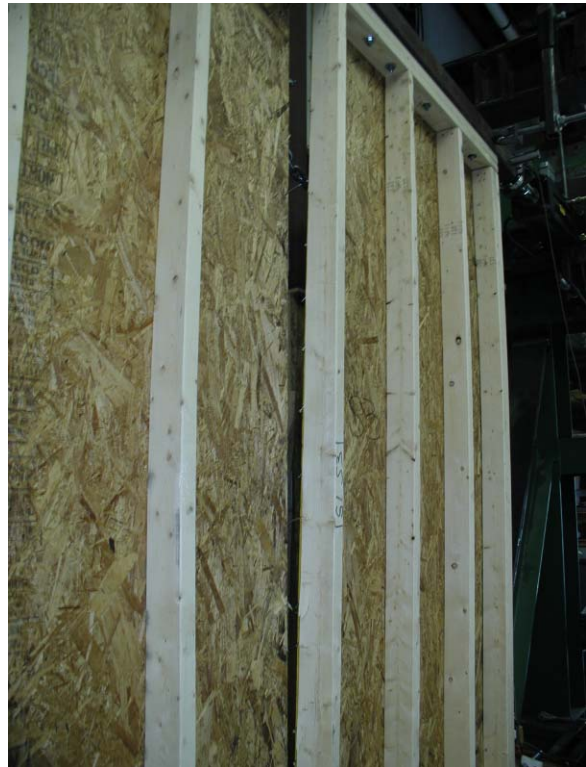
Separation of sheathing panel from framing after failure
