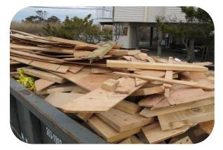
Using longer sheathing reduces the amount of waste at the jobsite. Less waste means fewer trips to the landfill.
